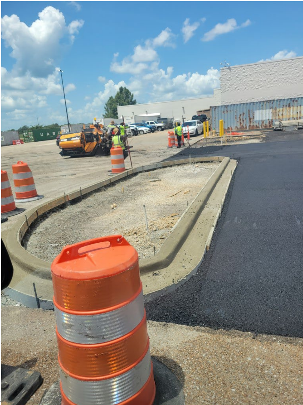
+ Curb has been installed. The subbase material has not been removed.
