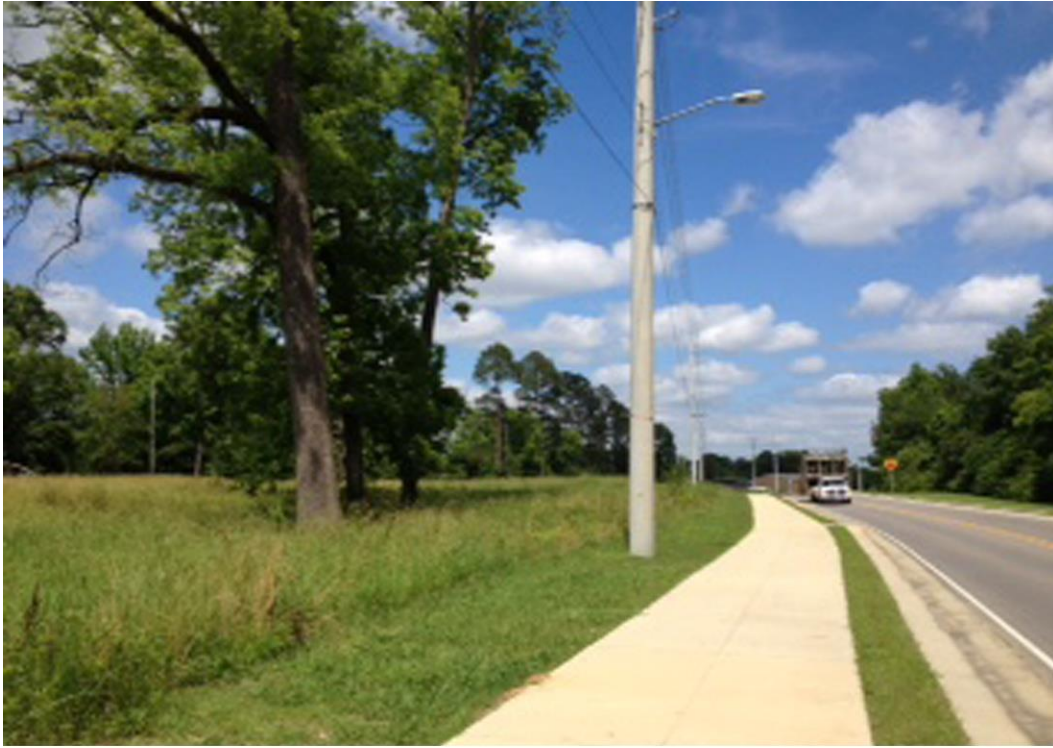
View looking east down Garrard Road
