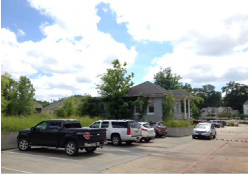
View looking southwest at subject property
