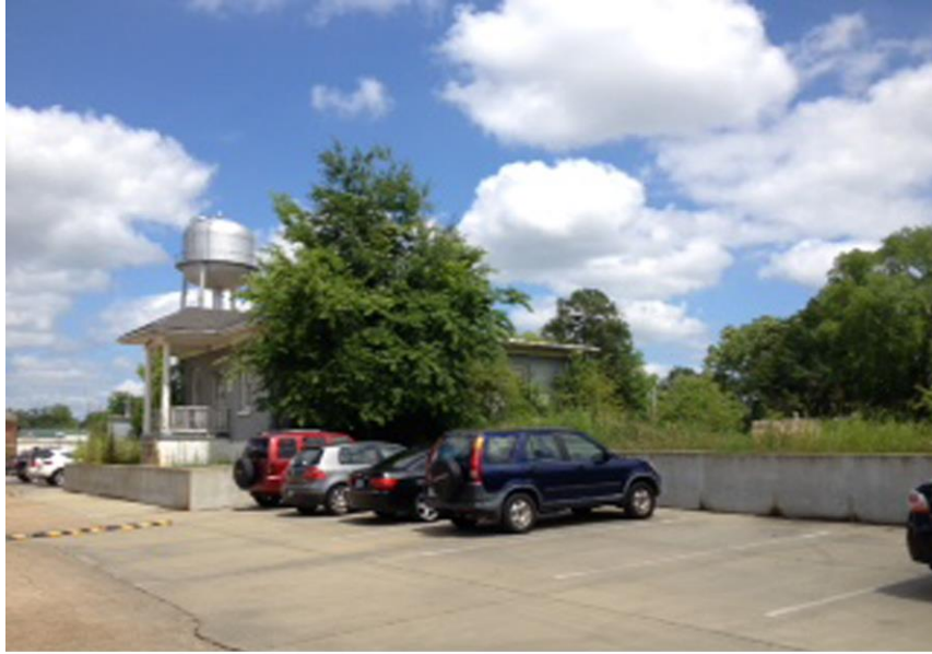
View looking southeast at subject property
