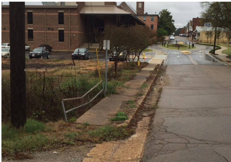
View of existing sidewalks along South Lafayette Street
