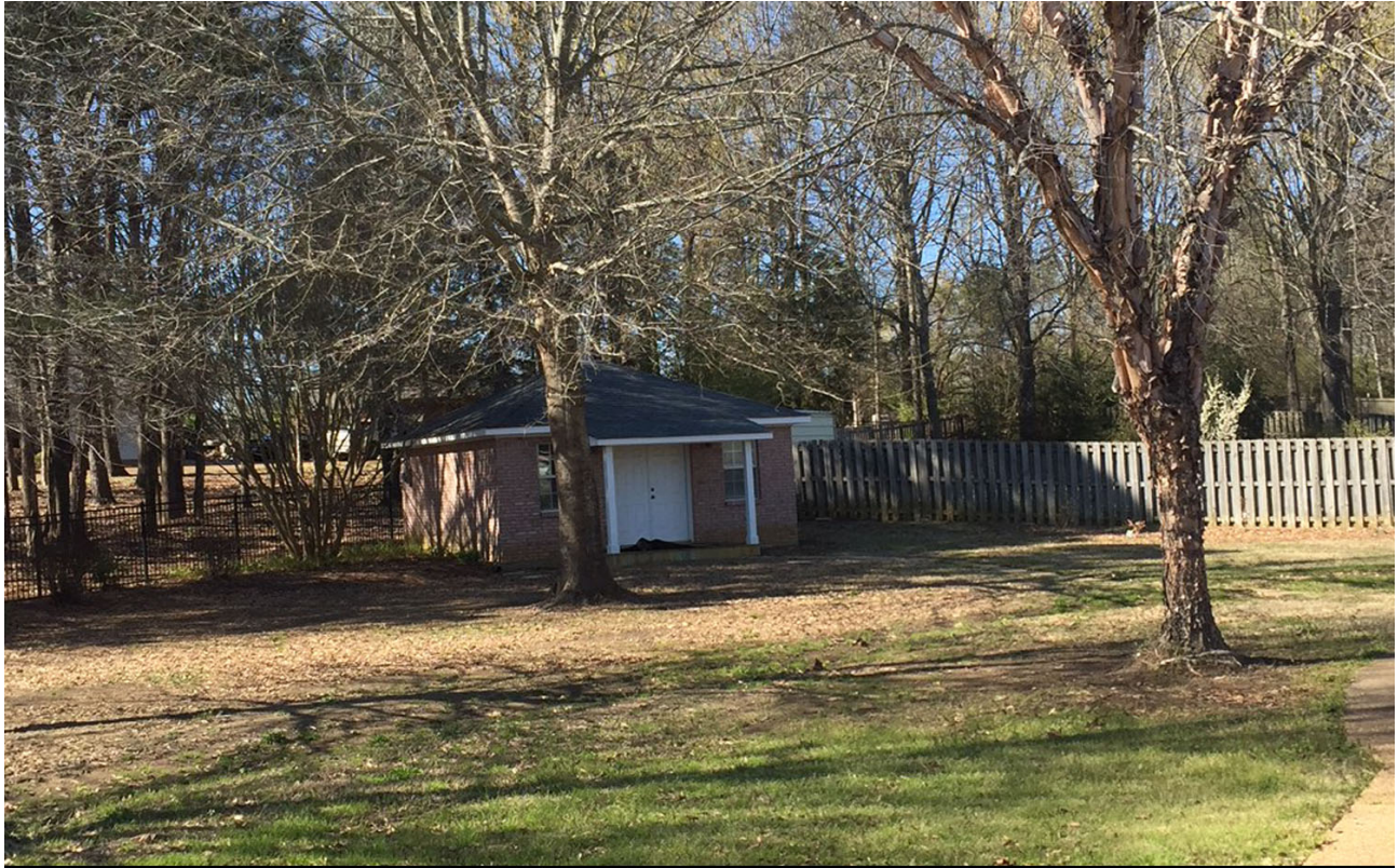
View of existing structure
