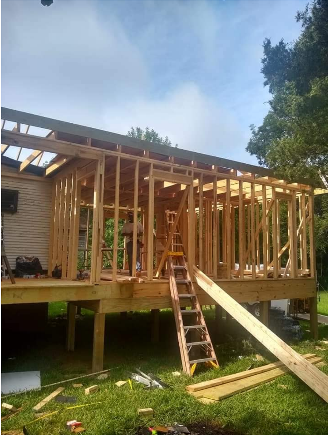
Attachment 5- Construction of dwelling unit #3
