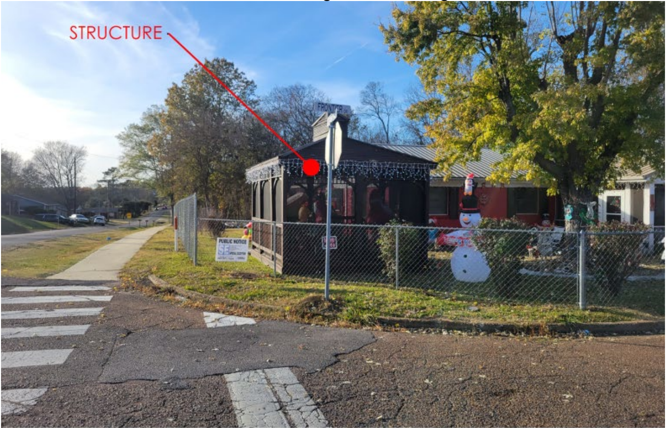
Attachment 4- Images of the Existing Structure
