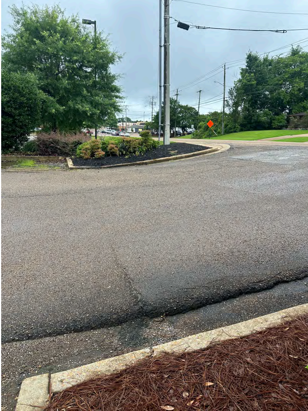
View of Temporary Easement Area from North Looking South
