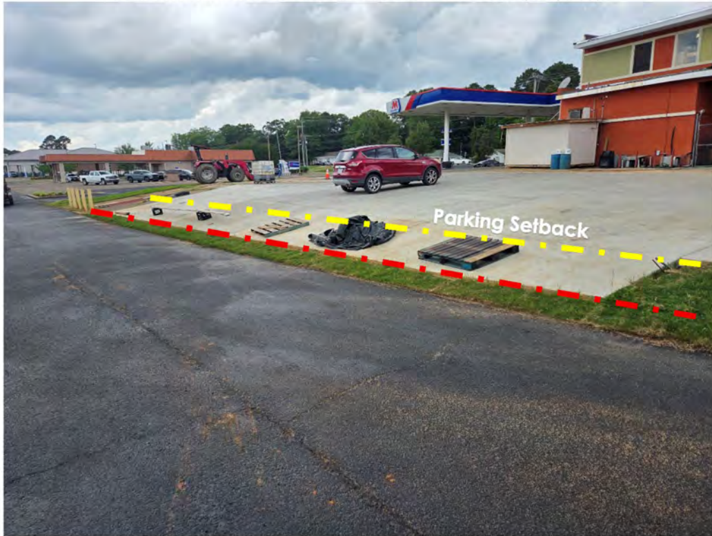
Pavement removed from Middleton Court property
