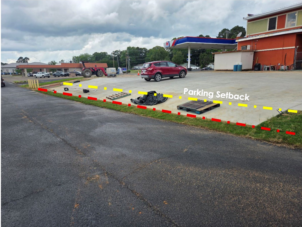
Pavement removed from Middleton Court property
