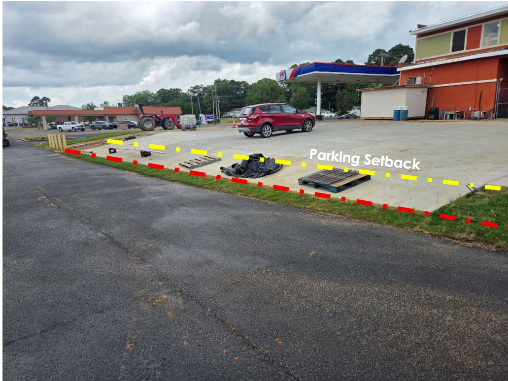
Pavement removed from Middleton Court property
